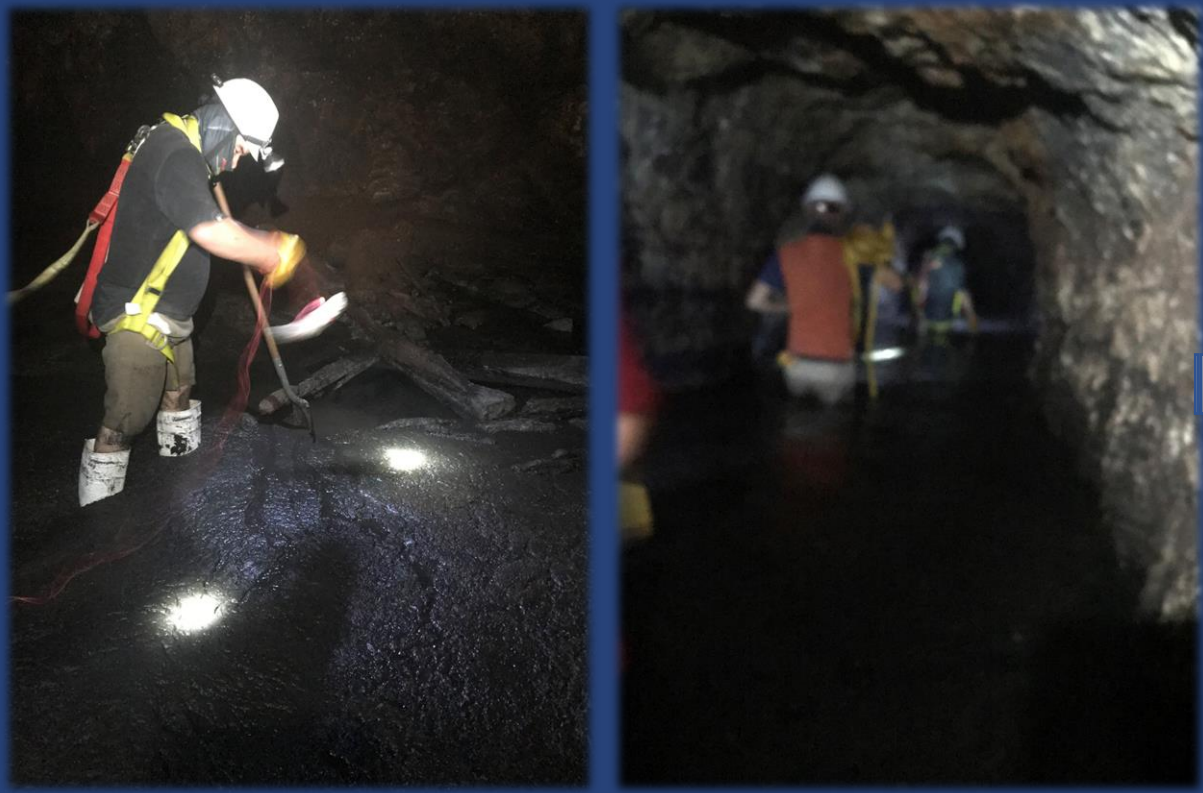
Accessing the haulage level towards the El Tirito shaft Significant amount of water and guano measuring 1 m high
